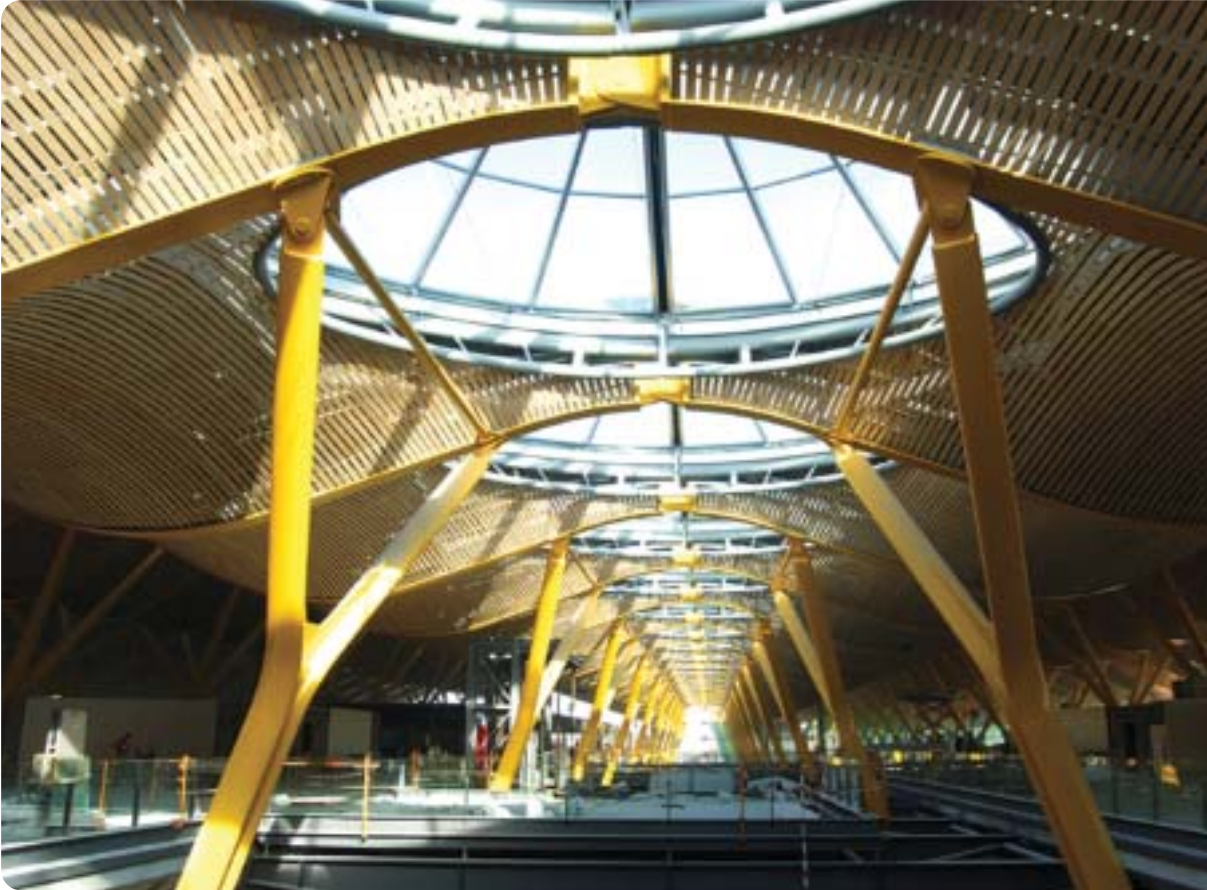
Roof of Barajas Airport Terminal. Madrid
