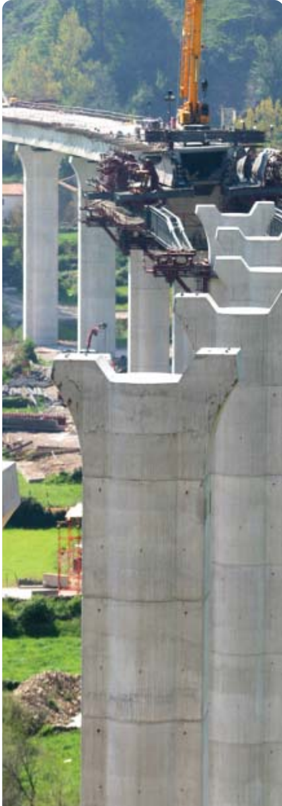
Pedredo Viaduct. Cantabria-La Meseta Dual Carriageway
