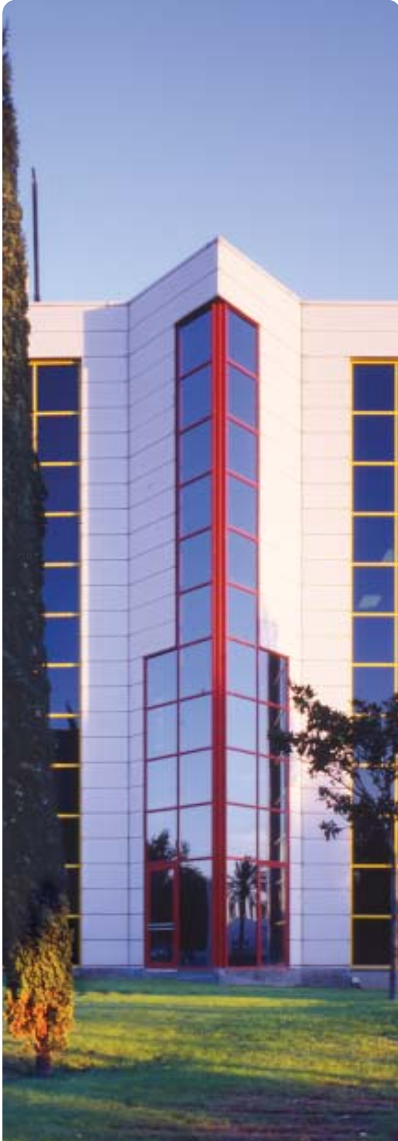
Muntadas I Building. Barcelona
