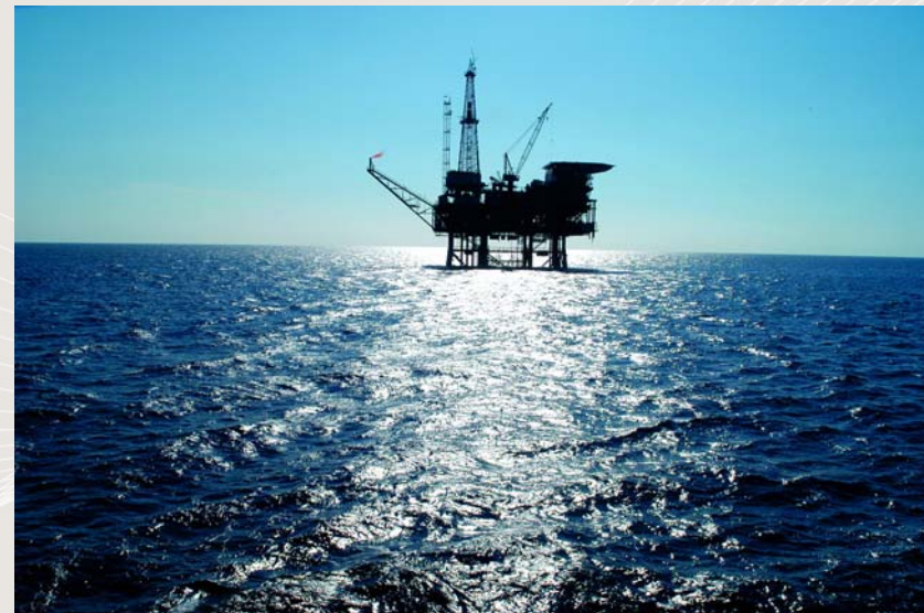
Casablanca Oil Platform, Tarragona. Spain
