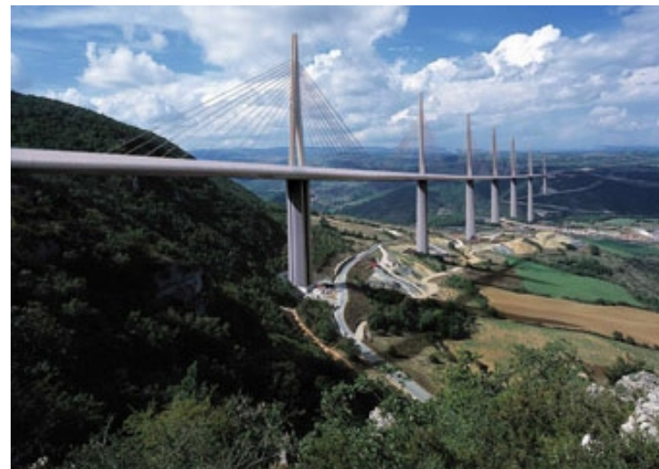
Millau Viaduct. France
