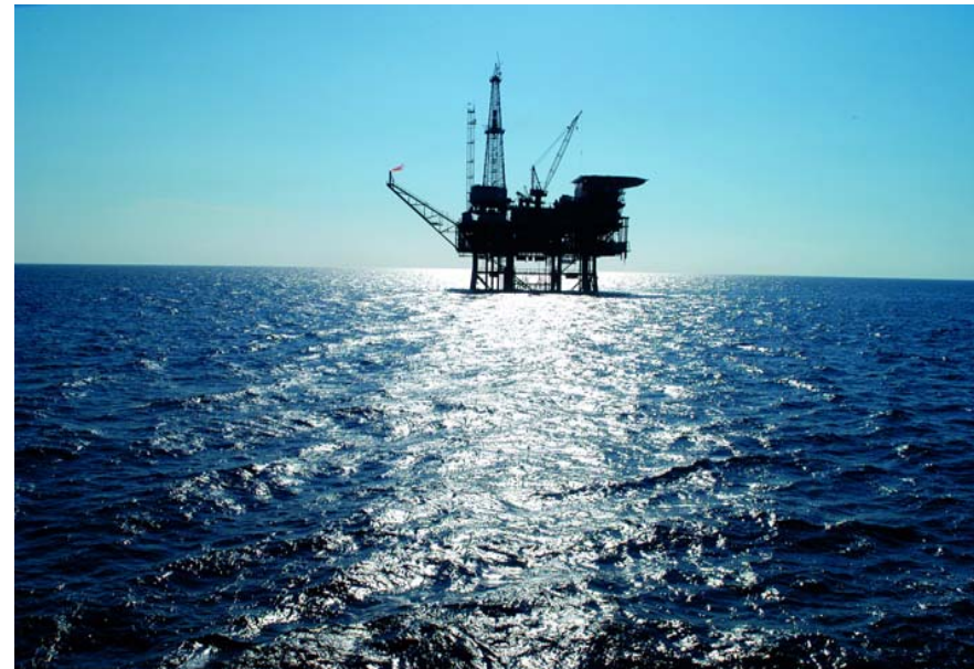
Casablanca Oil Platform, Tarragona. Spain
