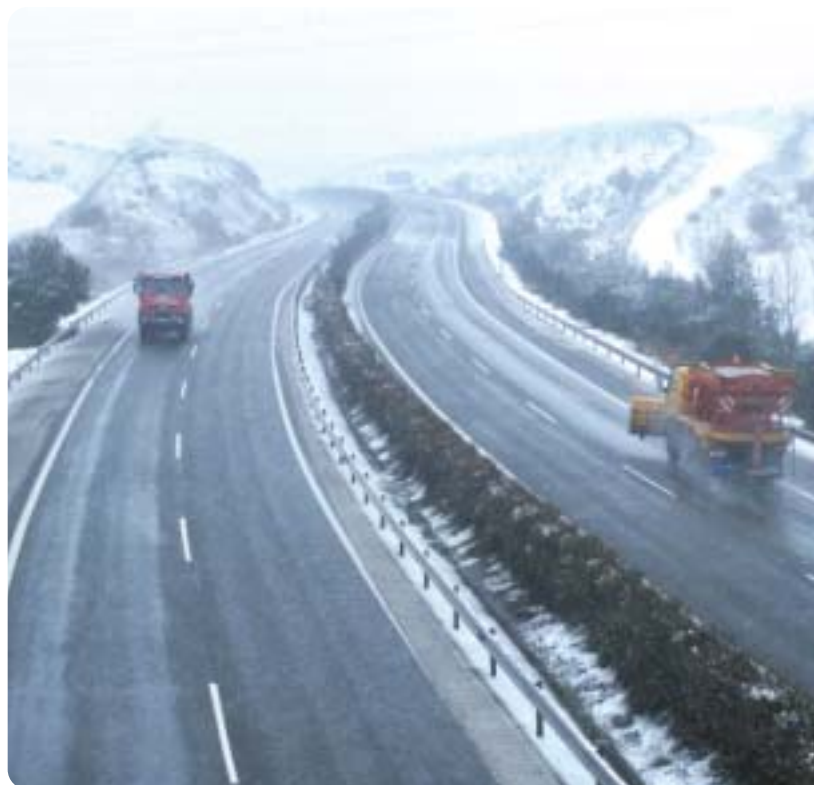
Road Maintenance. Audenasa
