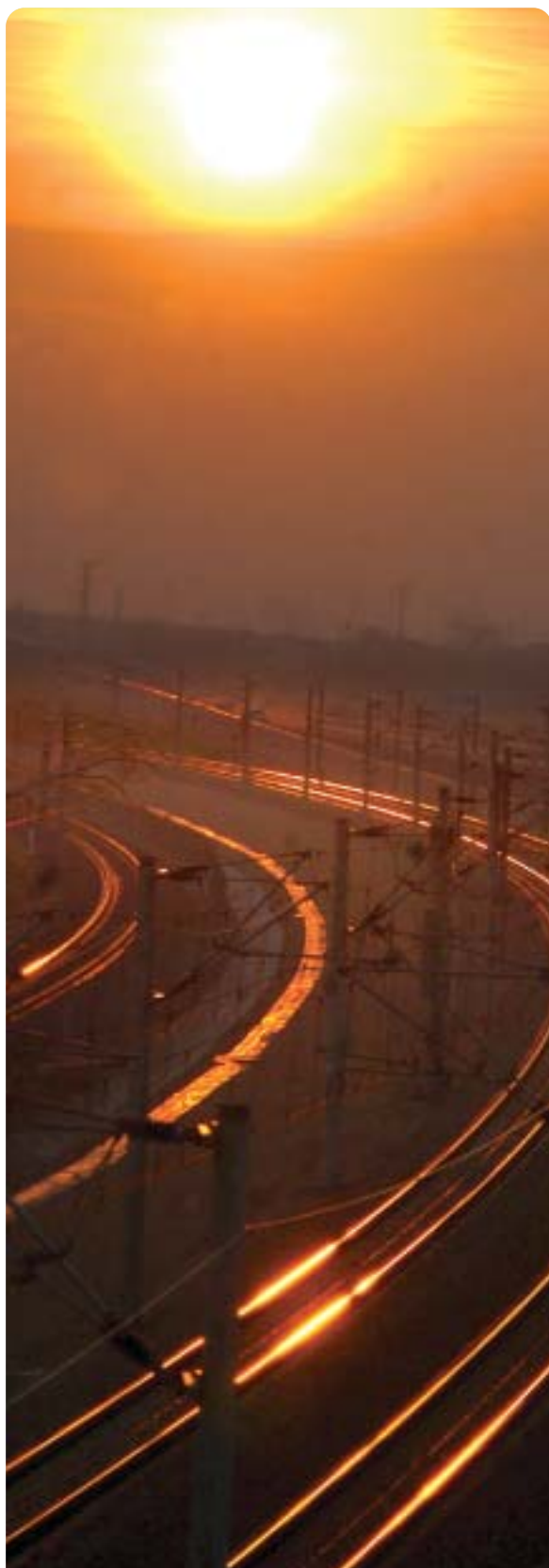
Cordoba-Malaga High-speed Link
