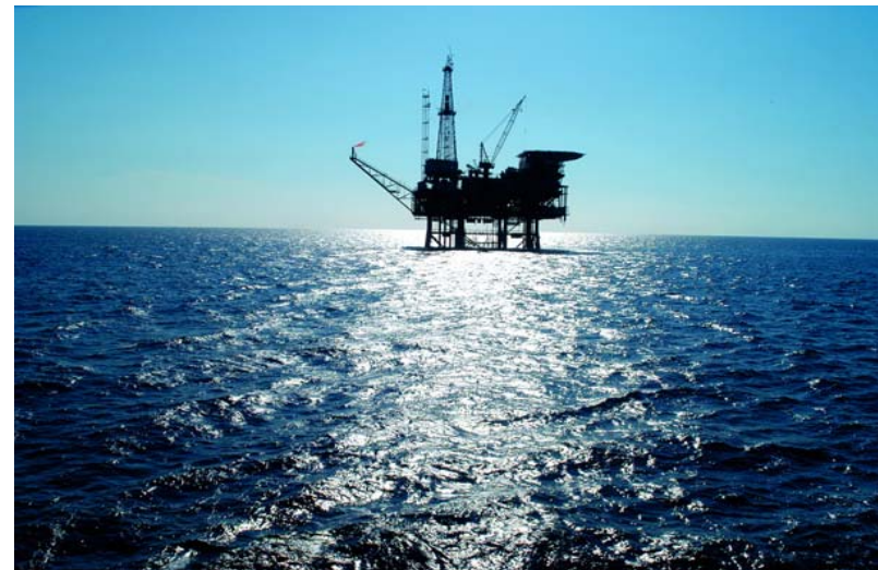
Offshore platform Casablanca, Tarragona. Spain
