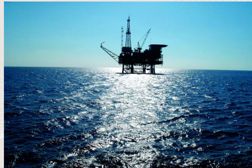
Casablanca Oil Platform, Tarragona. Spain
